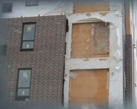
Traditional building wraps rely on fabrics and plastics which can tear and puncture.
