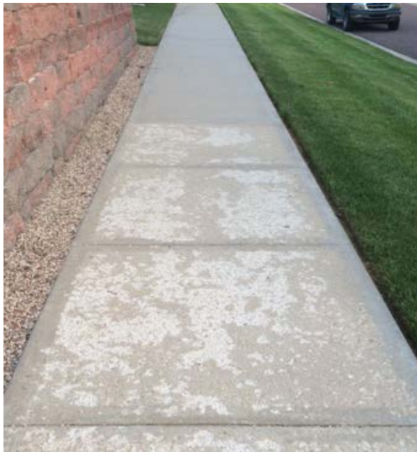
The dramatic difference between untreated surfaces (at bottom) and those treated with Salt Protector Plus™ WB (at top) is clearly shown above.
