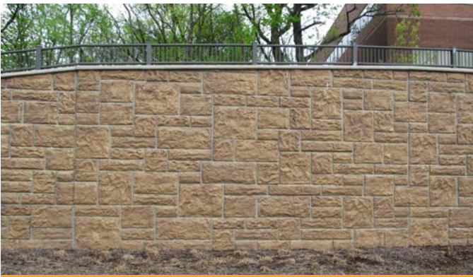
D.O.T. and Sound Barrier Walls
